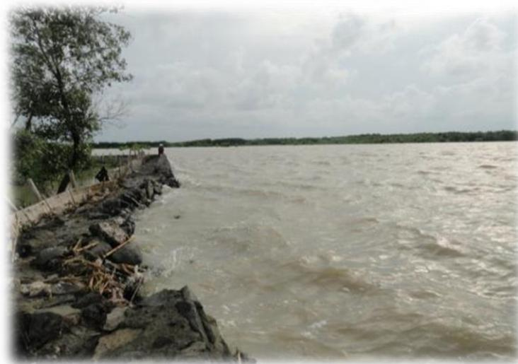
Waves reflect on hard structures, increasing eroding force
