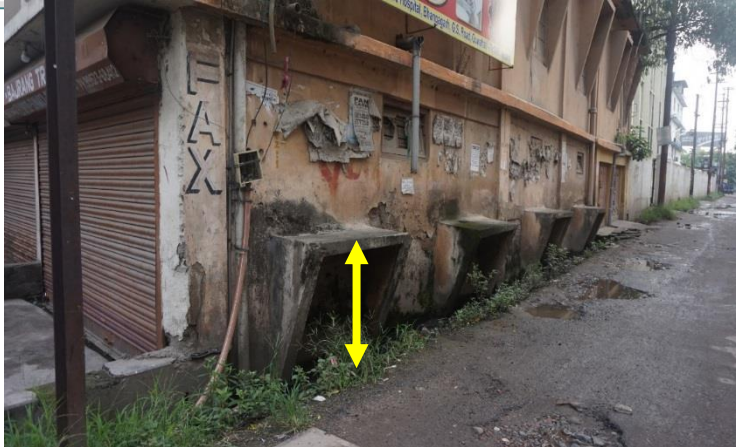
Building settled till sill level under action of flood water
