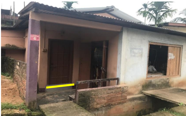
Building's settled till plinth level under action of flood water
