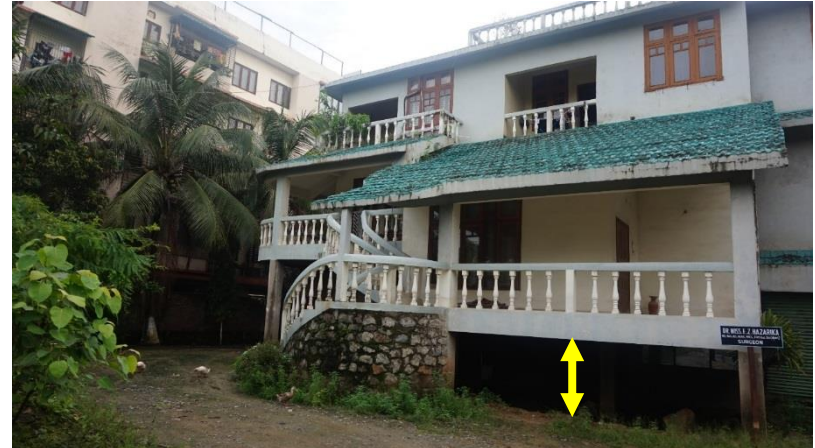
Building basement filled with mud brought by flood water
