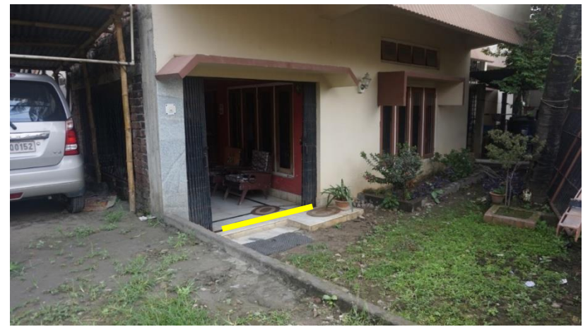
Building's settled till plinth level under action of flood water
